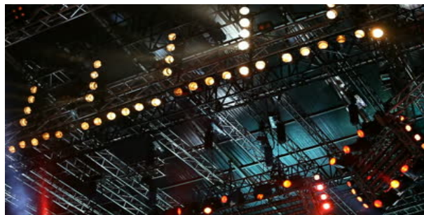
Figure 3.1: Complex Stage Lighting System
